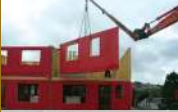
Erection of Timber Frame Structure at Beechgrove, Dromore
